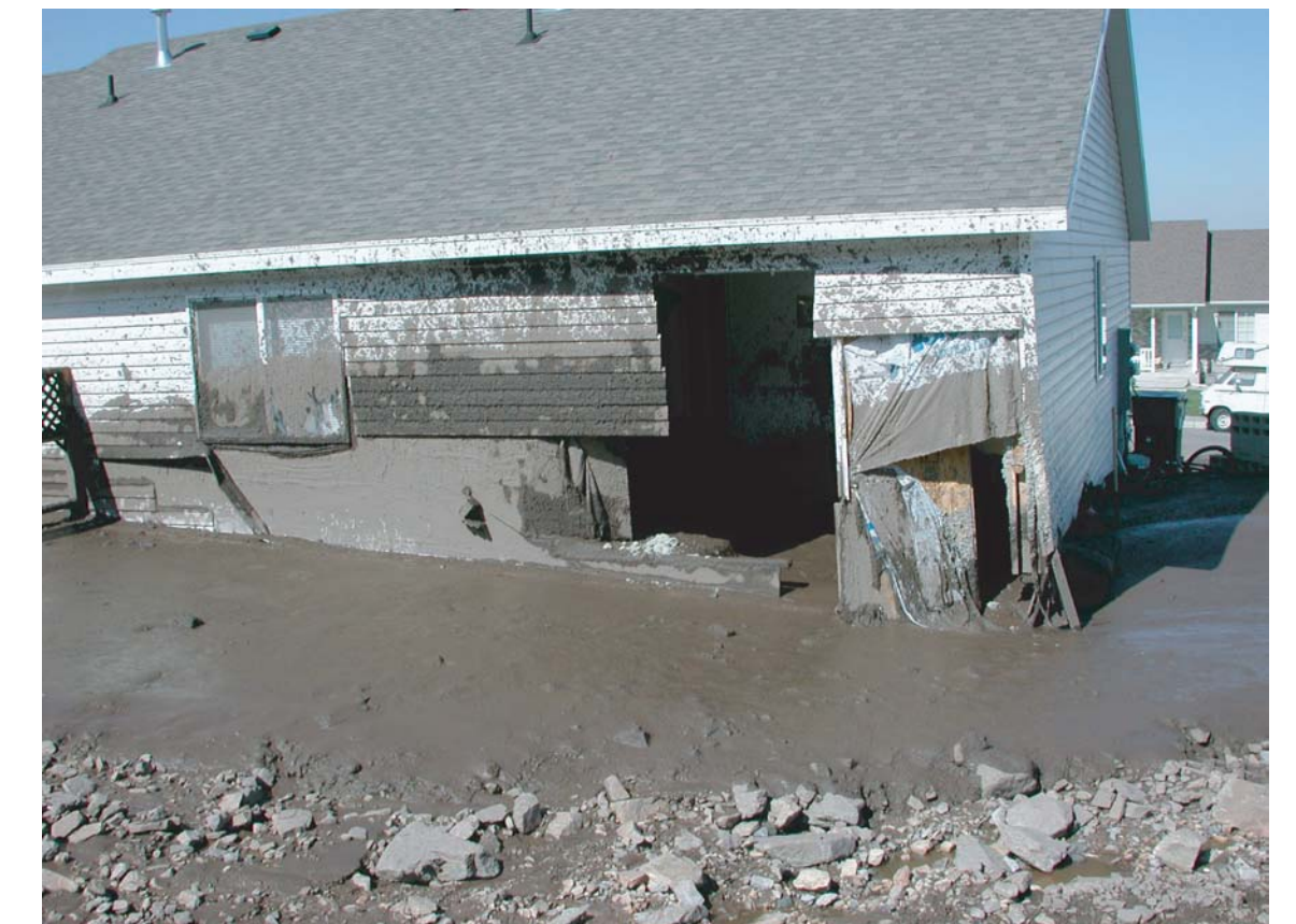
The September 12, 2002 debris flow broke through the back wall of this house on Peach Street in Santaquin (Utah Geological Survey photo).
