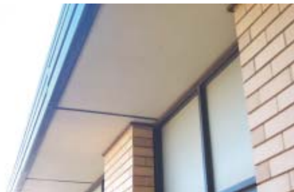
Promat's Promatec calcium silicate board material incorporated into eave linings on a home for construction in a bushfire prone area.
