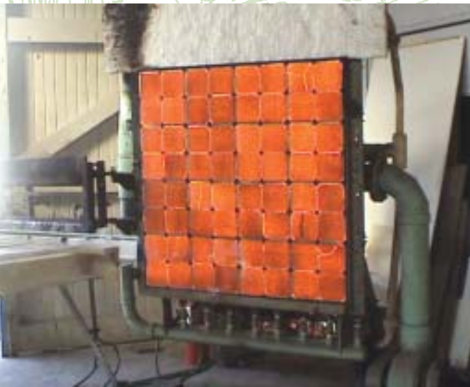
Laserlite clad timber framed pergola construction under bushfire fire test using a full scale radiant heat exposure panel
