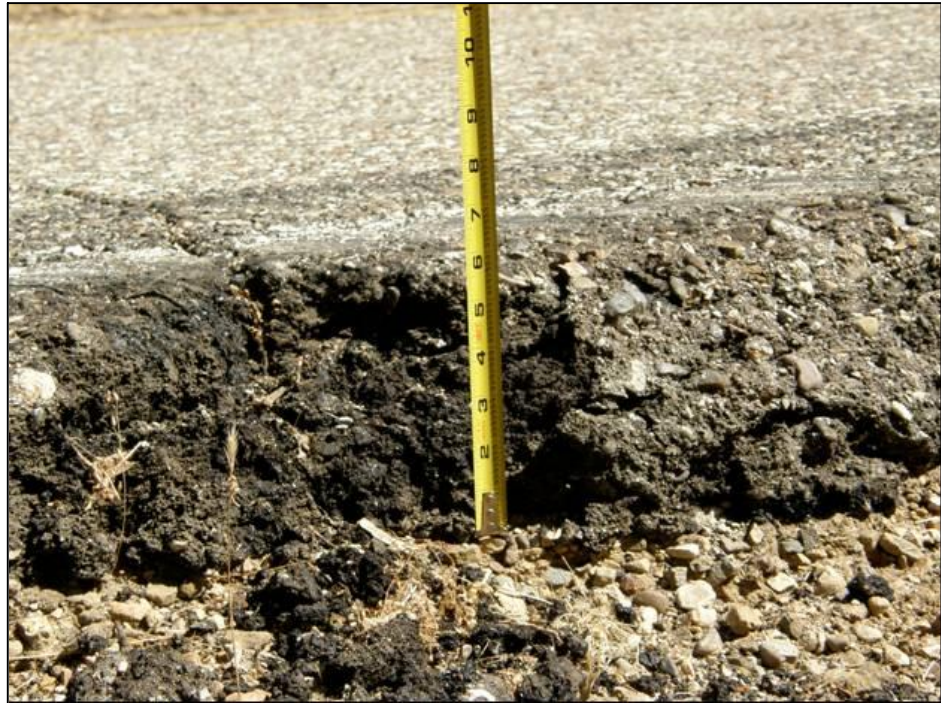
Fig 3 – Asphalt thickness and road edge where Engine 56's rear dual tires went off Vasquez Road.
