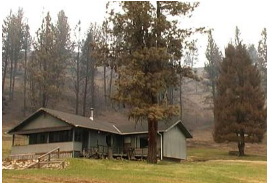
This well-prepared home survived a hot crown fire that passed nearby. Credit: Utah State University Extension.
