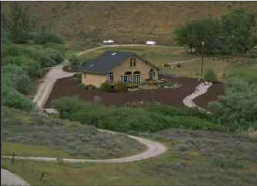
A narrow “home ignitability zone” determines whether a home will burn.
