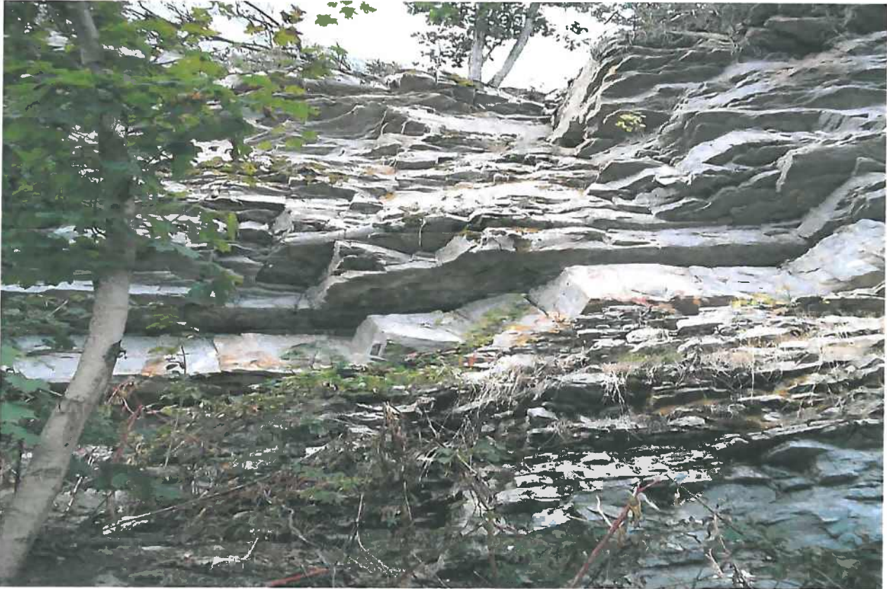
Rocky bluff that snag rolled over and struck employee.
