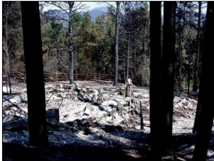
Photo 4—The unconsumed, moderately scorched tree canopy along with the remaining wood rail fence indicate that this home was exposed to a low intensity surface fire. The high intensity wildfire burned on the hills in the background.
