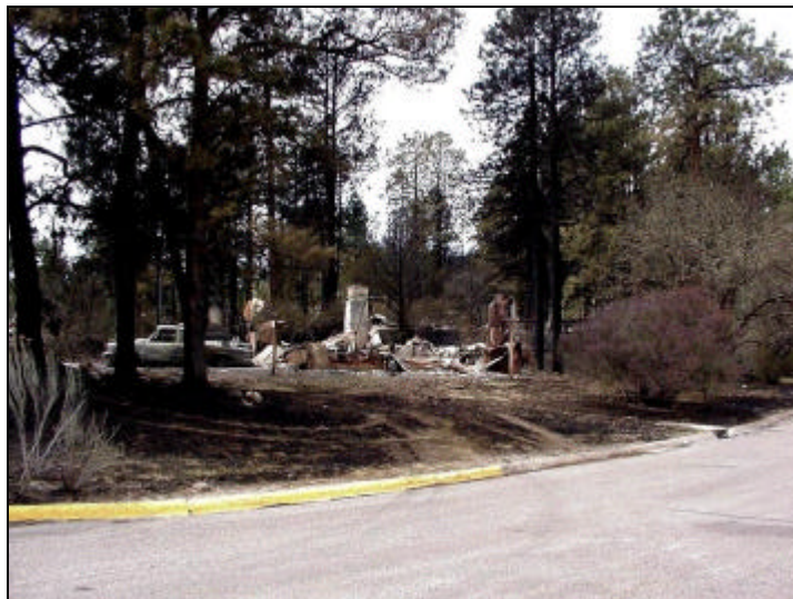
Photo 5—This totally destroyed home was within the residential area. A road separated it from other burning vegetation and homes. The unconsumed vegetation with little scorch indicates that the fire intensity surrounding the home was low. This suggests that firebrands (burning embers from other fires) ignited the home directly and/or in adjacent flammable materials that spread to the home.
