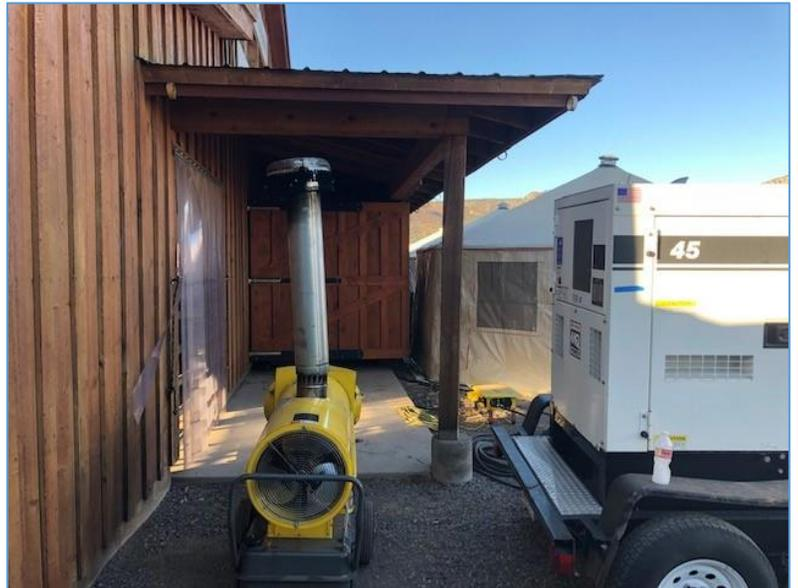
It was determined that because the (yellow) heating unit was placed next to a building with an overhanging roof, the unit's exhaust was trapped and cycled back into the unit's air intake, which was then pumped into the Medical Unit yurt with warm air. The yurt is seen on right in the distance; the generator is on right in foreground.
