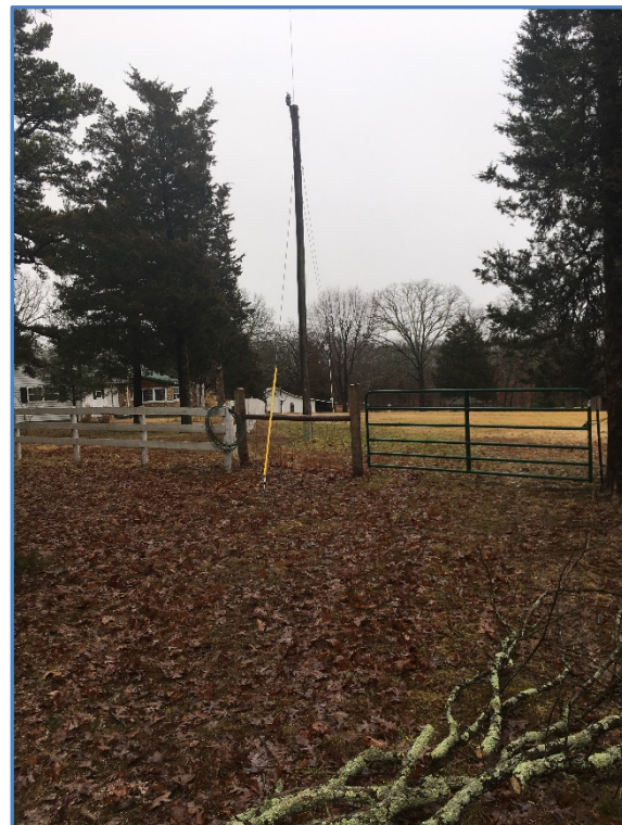
The top of the fallen tree that covered the powerline.
