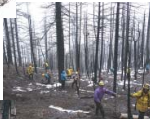
Log erosion barriers near Lemon Dam
